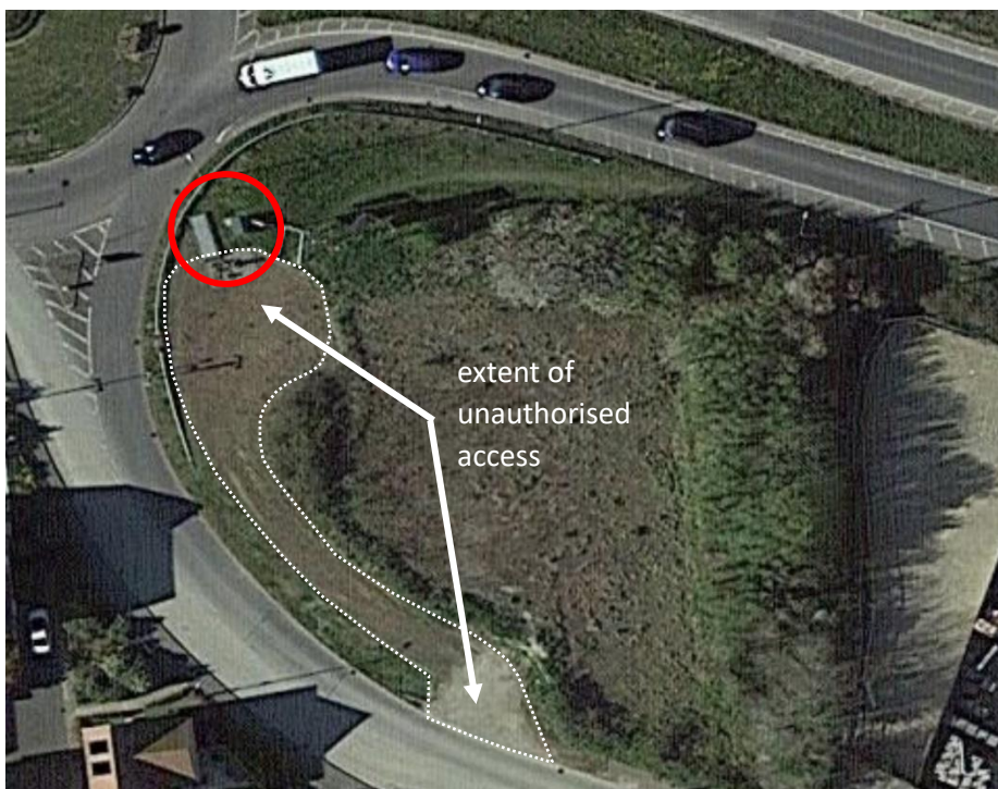
figures 32: The Anglian Water pumping plant
